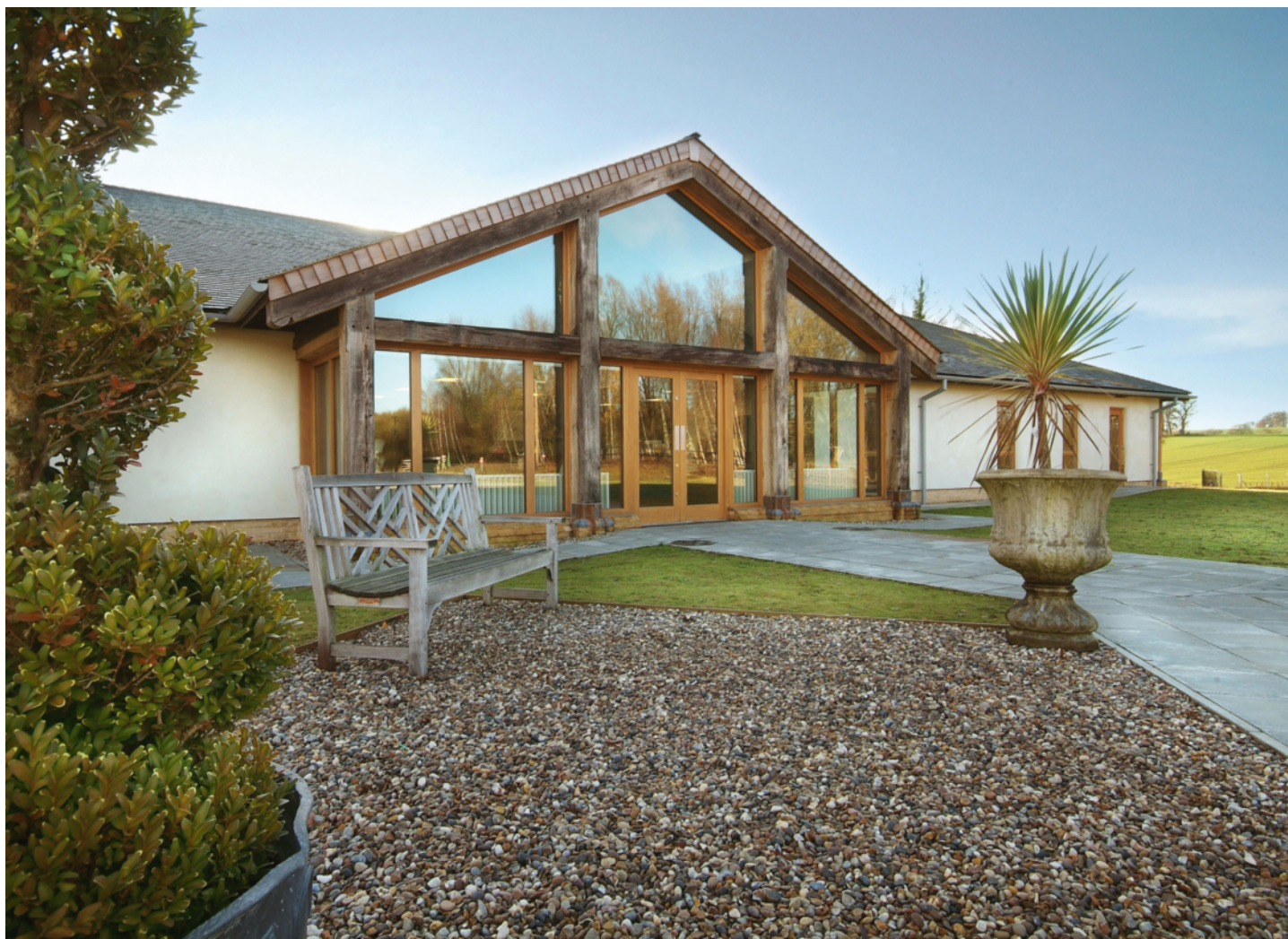
A new future with ancient materials: the lime-rendered, straw-bale headquarters of Sworders of Stansted Mountfitchet in Essex
